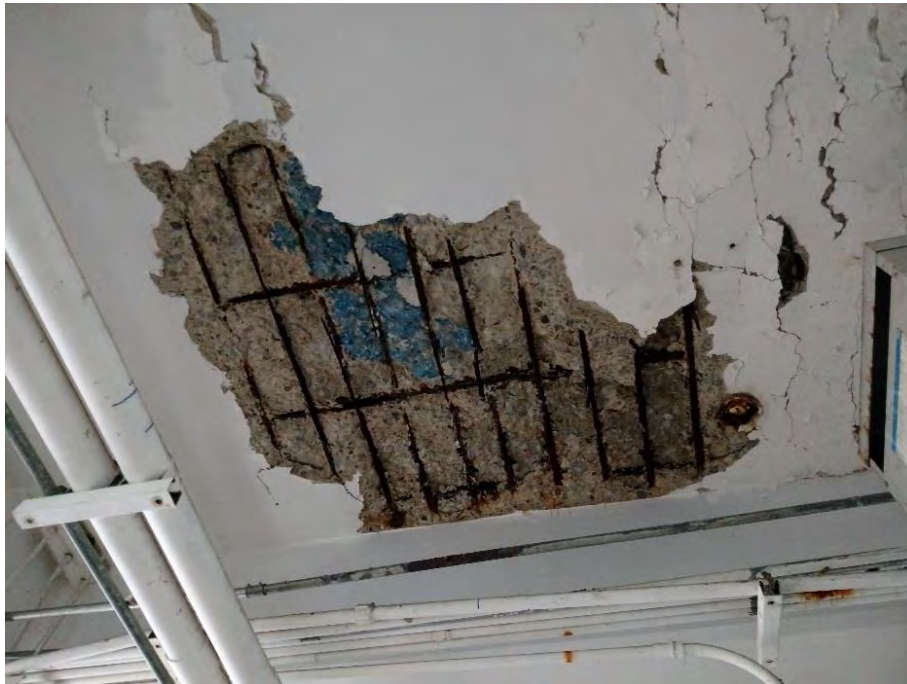
Figure 25 Water Treatment Plant control building deteriorated roof slabs
